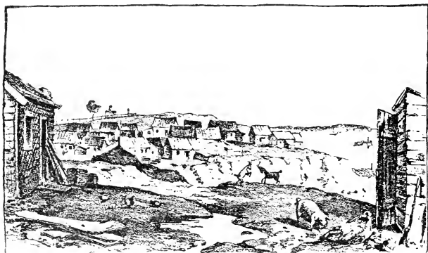
OLD SQUATTER SETTLEMENT ON THE CENTRAL PARK SITE.
